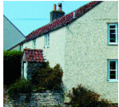
Colour - timber was usually painted in soft, natural pigments and was typically white or cream. Ironwork was usually finished in white or black. Render was usually left natural or cream coloured (originally lime washed). Agricultural buildings were left naturally coloured
