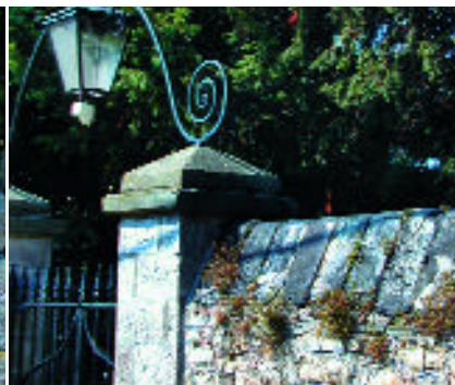
Boundary wall - irregular stone walls form edges to gardens and building boundaries, usually topped by a distinctive 'cock and hen' random stone capping, or occasionally stone copings with wrought iron railings above. The grander the building, the more elaborate the boundary treatment. The walls around St Mary's Church are topped with unusual black slag block copings, a by-product of the 18 th century brass industry around Bristol
