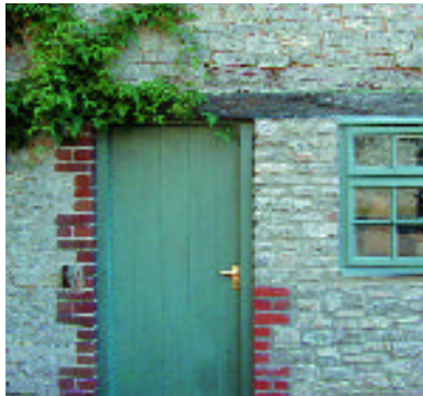
Doors - usually unprotected from rain, solid timber panelled or planked and painted. If money allowed, a timber and glass porch was added to provide cover and express the individuality of the owner
