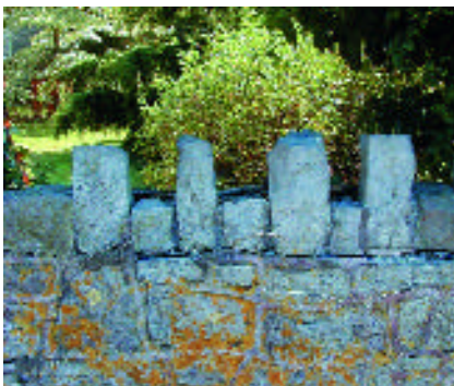
Boundary wall - irregular stone walls form edges to gardens and building boundaries, usually topped by a distinctive 'cock and hen' random stone capping, or occasionally stone copings with wrought iron railings above. The grander the building, the more elaborate the boundary treatment. The walls around St Mary's Church are topped with unusual black slag block copings, a by-product of the 18 th century brass industry around Bristol
