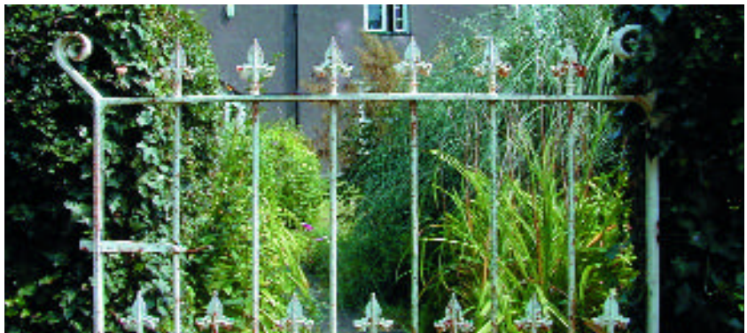
Ironwork - mostly removed in World War II. Originally, many boundary frontages were designed to incorporate wrought iron railings and gates. The more refined the building the more likely that expensive ironwork was a feature, although even unassuming buildings would often have an iron gate. Ironwork was typically simple in form and in keeping with the style of building
