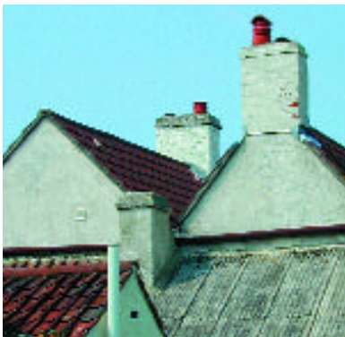
Chimneys - the ridge line was usually punctuated by simple rectangular stacks in brick or stone topped by clay chimney pots
