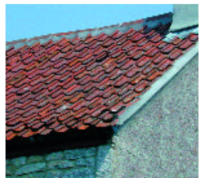
Roof / wall junctions - typically unadorned with little or no eaves overhang or timber fascia. Usually the roof gable has no bargeboard
